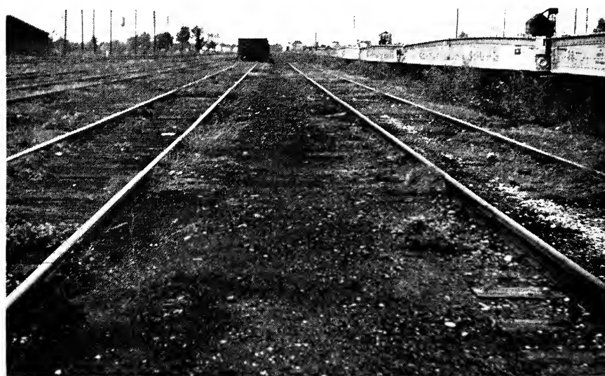
Fig. 3—Treated in June 1954 with 44 lb of Dalapon and 2 lb of 2, 4-D per acre. Photo taken in October 1954.
